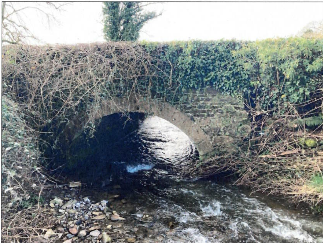
Plate 3-24. View of stone arched bridge crossing an EPA mapped watercourse classified as Eroding upland river (FWI) along the Proposed Grid Connection underground cabling route.
